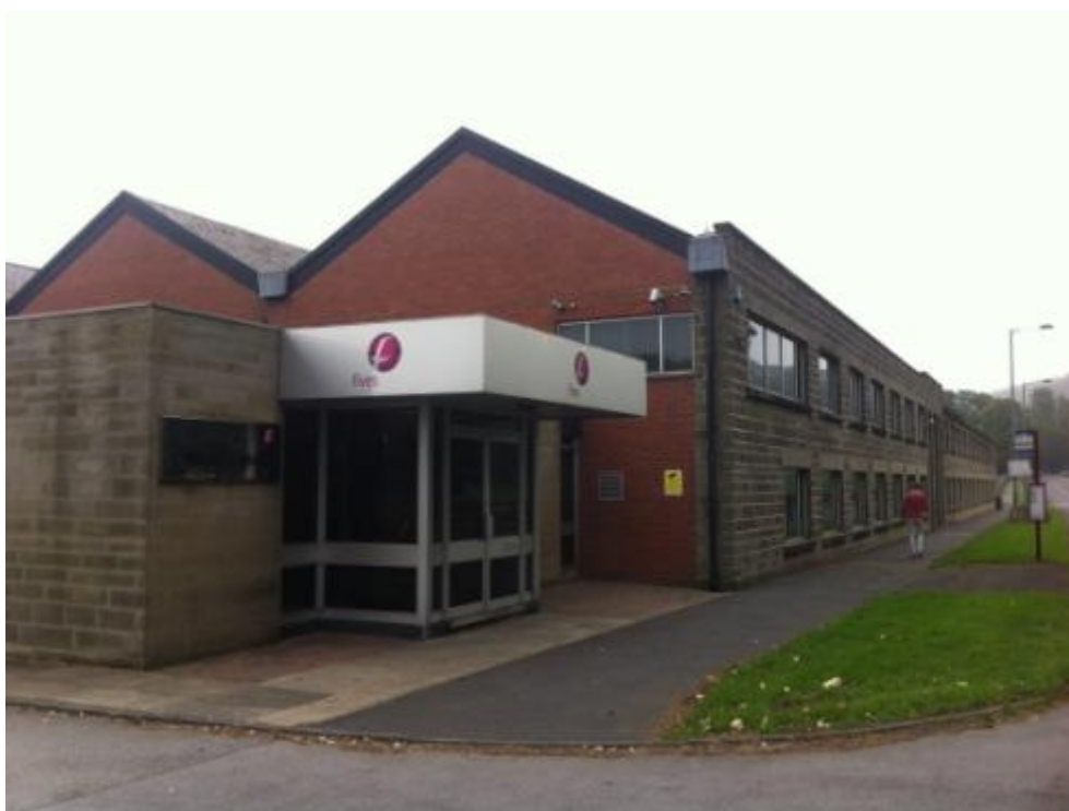
Eastbourne Works, Skipton Road, Eastburn
