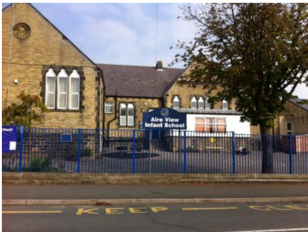
Aire View School, Silsden
